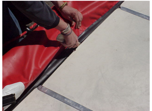
Step 6: Inflate using pump included to 6 PSI
